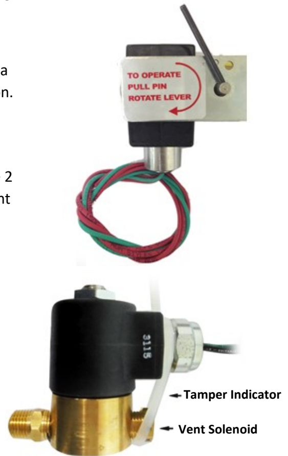
Figure 2—Electric Solenoid Tamper Seal
